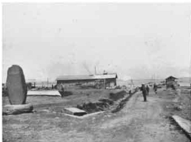
第 301 圖 大谷村大谷。津波前は此の邊一帶に住宅及納屋ありしも皆流失す。津波は写真左手の明治 29 年の海嘯記念碑の頂下 5 寸程迄届きたりと云ふ。此の邊津波の高さ平均海面より 4.5 米。(5 月 18 日 高橋操撮影) Fig. 301. Oya, Oya-mura The houses & cottages which stood before the tsunami were all washed away. The water reached a height of 15 cm beneath the top of the stone-monument (the monument of the tsunami of 1896) shown at the left of the photo. (Photo by R. Takahashi, May 18.)
