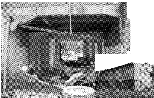
Fig.9 Damaged building in case of the 2004 Indian Ocean tsunami at 3.7 m flow depth.
