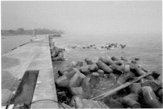
Fig.3 Erosion of armour layers in front of a caisson breakwater
